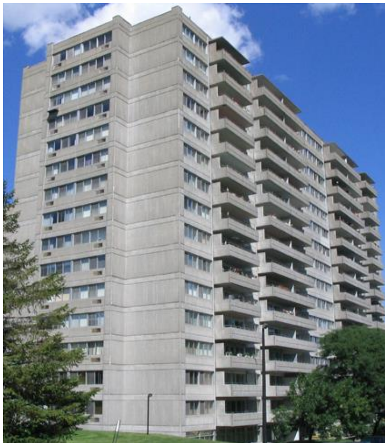
Manoir IV, view of the rear of the building
